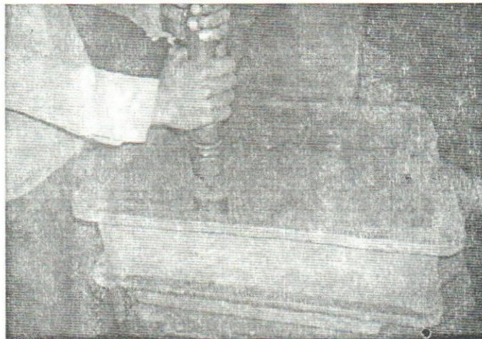
Figure 5.5: KIAZEN- Use of Pneumatic rammer
